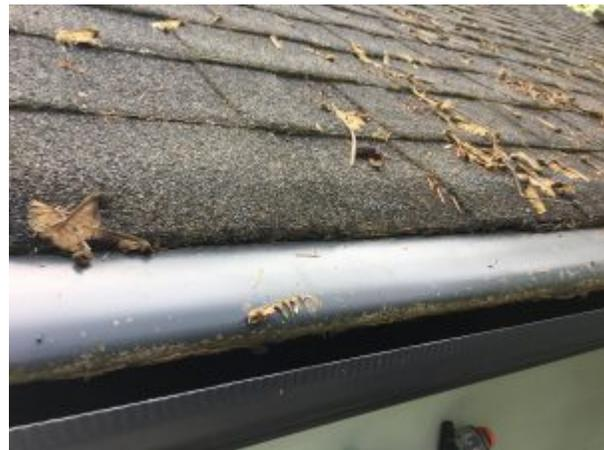
Figure 3. Gutter guards prevent the accumulation of biological debris in the gutters and rain barrels. Photograph courtesy of Dorothy Yee Leggett.
