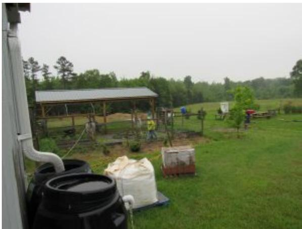
Figure 1. Typical garden rain barrel installation. Photograph courtesy of William McCaleb.
