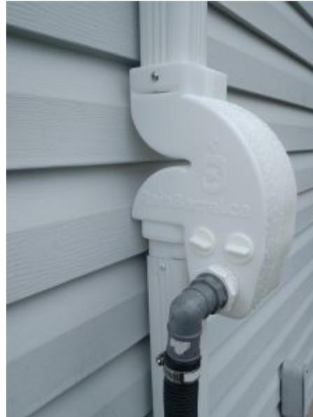
Figure 2. A diverter for protecting water quality in the barrel. Photograph courtesy of Mary-Jane Pilgrim.
